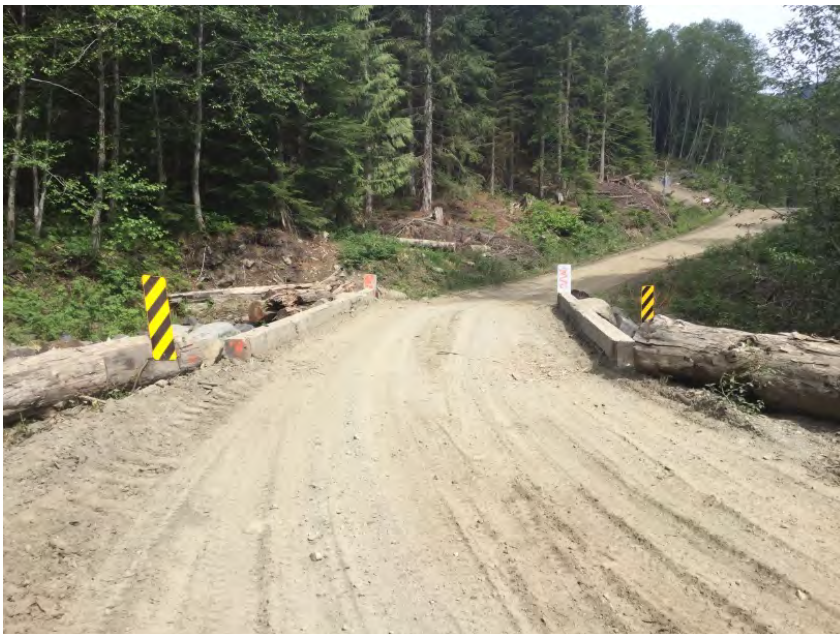
Approach from Right Bank when facing downstream
