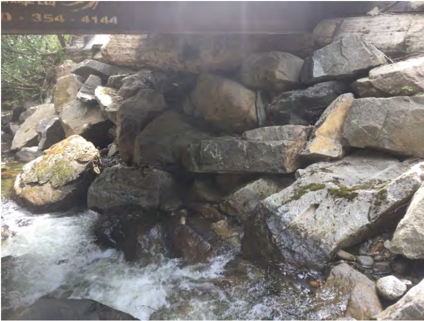
Right Bank Abutment when facing downstream
