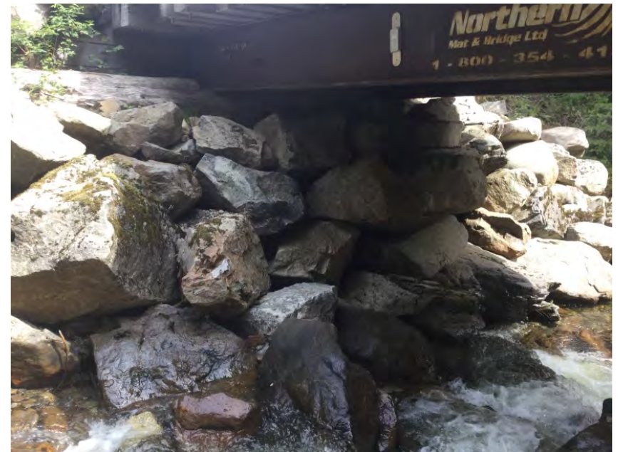
Left Bank Abutment when facing downstream
